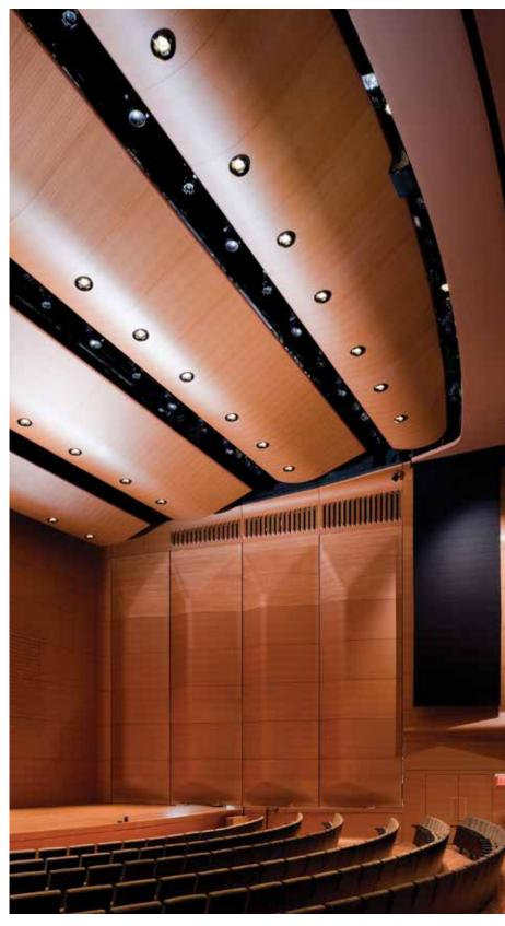
"We had especially tight clearances between the first reflector and the mounted concert lighting fixtures," states Rosenbaum, adding that 3-D modeling and evaluating mock-ups ensured this reflector would never clip or bang into any light fixtures. Praising the successful team effort, Rosenbaum states, "We all pushed each other to find an acceptable solution that would fit the available space."
